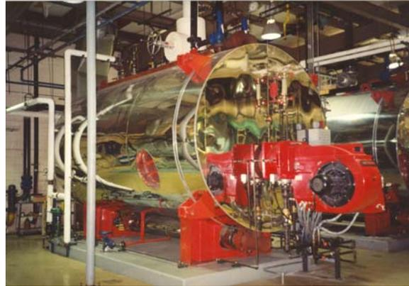
Three fire-tube steam boilers of advanced design at Tucson Medical Center
